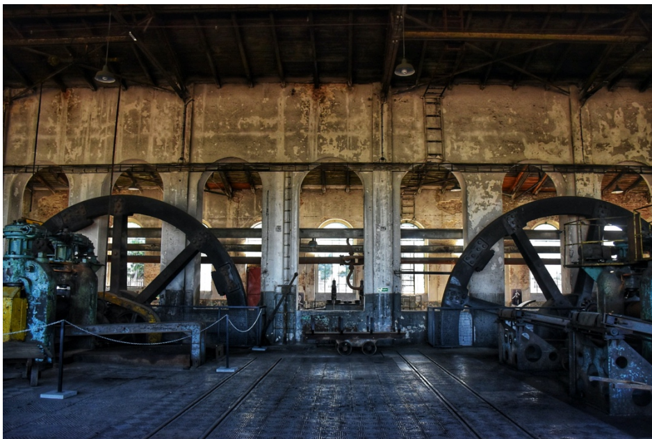
Fig. 3: The interior of the Zinc Rolling Mill Hall. in Katowice, view of flywheels from steam engines, currently the Museum of Zinc Metallurgy in Katowice, 2019. Source: P.Chodac
