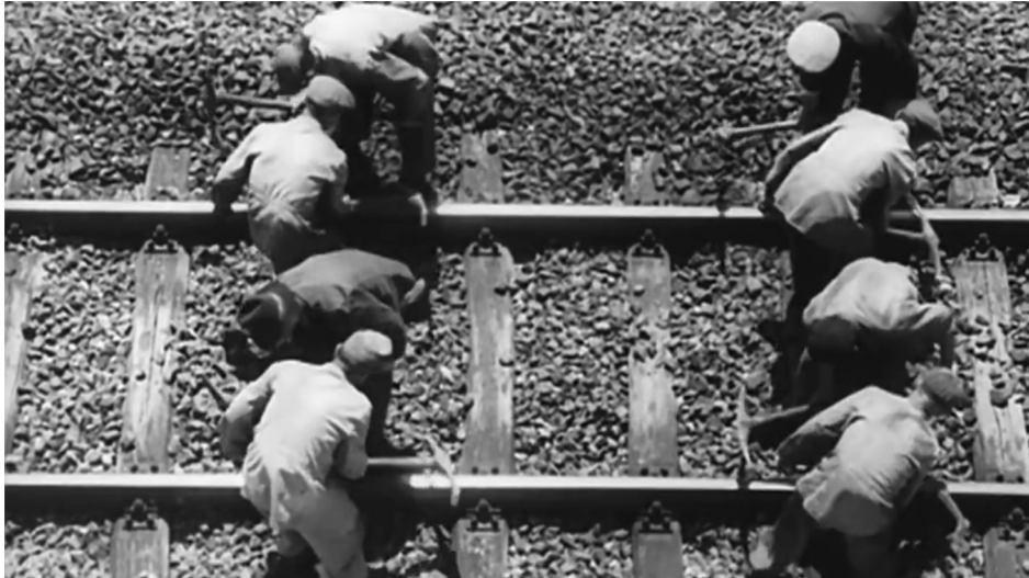
Fig. 10: Tamping the ballast (Source: MMA Youtube channel)
