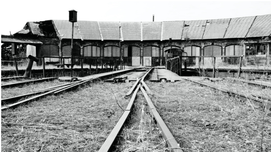
Fig.1: Marshalling yard, Novi Sad, 2021. Source: Antal Szilárd
