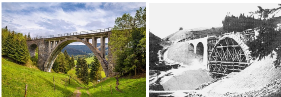
Fig. 3: Technological scientific and social values are represented by the 22m-high and 86m-long Telgártsky viaduct, which was the first articulated arch structure made of reinforced concrete on the ČSD lines. Source: Ing. Jozef Pilko
