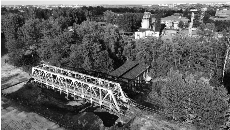
Fig 3: Sand railway bridge in “Wieczorek” coal mine, 2024. Source: Maciej Mądry
